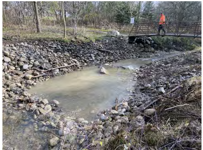
Downstream of the bridge (after): The bank has been shaped to a gentler slope and stone with filter cloth underlay was added.
