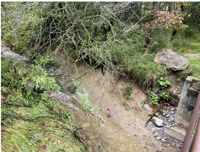
Upstream of the bridge (before): Bank erosion was undercutting trees and impacting the bridge abutment.
