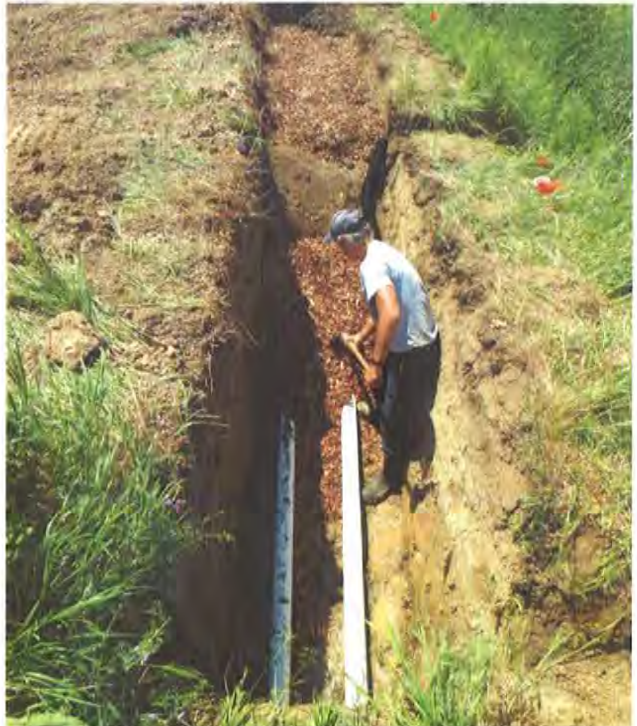
Staff install a woodchip biofilter.
